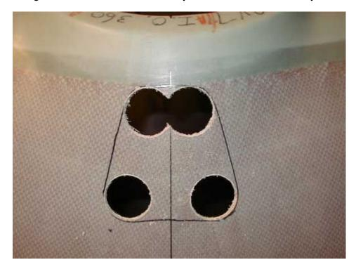
Once you've got the corners done, rough out the opening with a hacksaw blade or jig saw. It is nice to cut this opening on an angle that will follow the angle of airflow.
