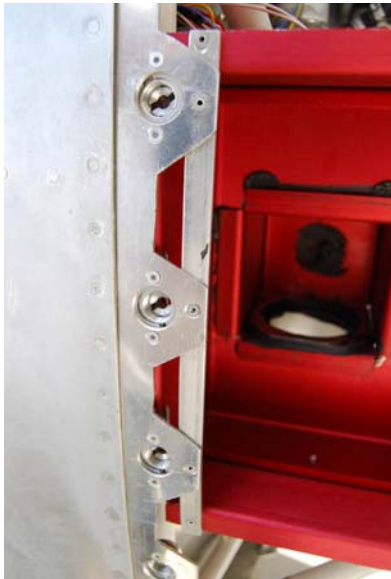
Using a strap to secure the frame.
