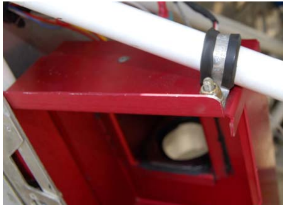
Using Adel clamps to secure the frame.
