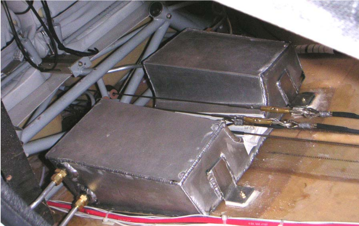
Under-floor common header tank installed. Note cable pass-thru channel.
